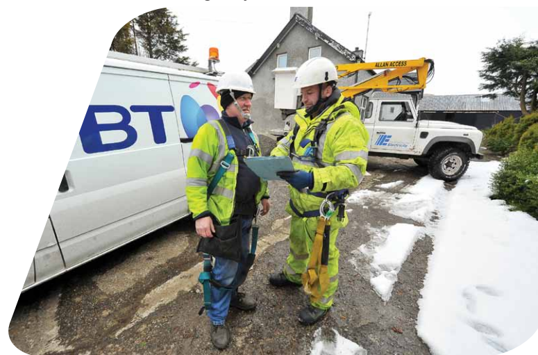
NIE & BT working together following the March snow storm
