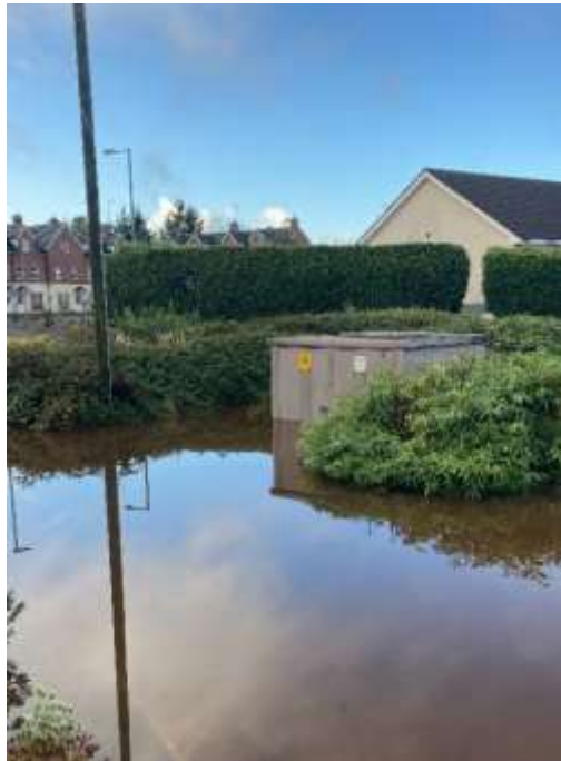
SUBSTATION FLOODING
