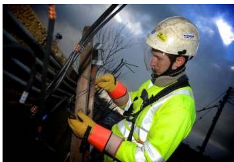
NIE apprentice at NIE's overhead lines training centre at Campsie.
